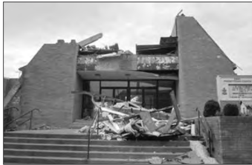
First Presbyterian Church, Cambridge, Ohio, following straight line winds in 2012. Photo by Pauline Albrecht, NRT.
